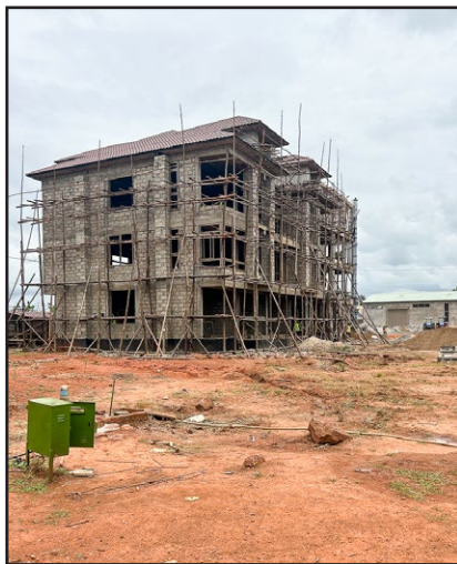
The administrative and STEM center building at the AMC Farm in Uganda under construction, October 2023. Photo by Molly Levine
